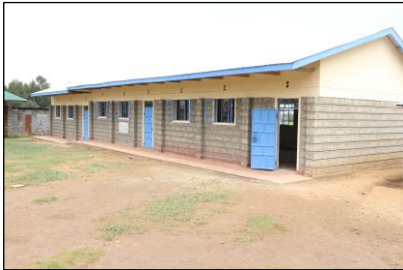
New, completed classroom building for Kahuria Primary School.
