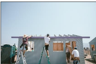
A visiting team is at work constructing a home.
